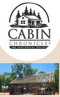
All of our barn's roof rafters are now installed. The next step in the building process will be the installation of a metal roof. Tuepker Bros. will be beginning that work soon. In the meantime, we are still in need of additional barn wood. If anyone has "leads" on either barn wood, or a barn to be razed, please get in touch with a member of the IHS. Your help will be greatly appreciated.
