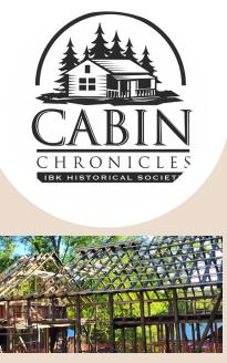
Note from the photo above that all but two of the roof's rafters are now in place. What's most amazing about this is the fact that ALL of the trusses were positioned without the use of any mechanical means other than ropes and pulleys. Our volunteers, using patience, determination, brawn, and lots of thought, were able to get the job done. A big thank you to our volunteers for a job well done. Because of limited space, the last two will be installed with the use of a "boom" type crane.
