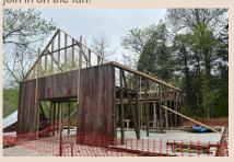
The latest photo (above) shows the recent placement of both gamble ends of the barn. Our crew has been working tirelessly, and are far ahead of schedule. Next will be the difficult task of placing the roof rafters. This portion of the reconstruction is likely to take quite a bit of patience, time, and planning. If you haven't seen the barn work, stop by on Saturday, May 11 at our Discovery Day Open House.
